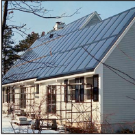
House, Belmont, Massachusetts Solar House, 1974
