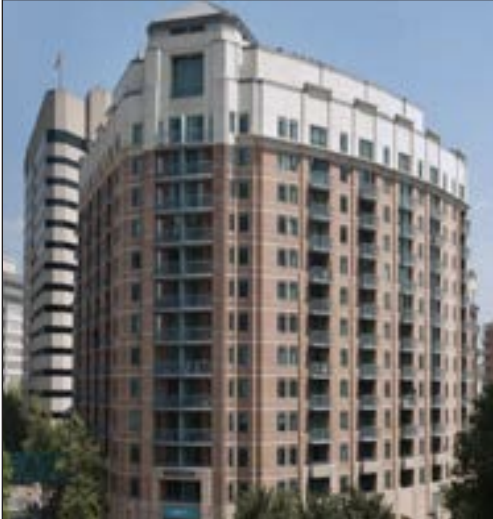
The Metropolitan, Bethesda, Maryland, (Completed)
